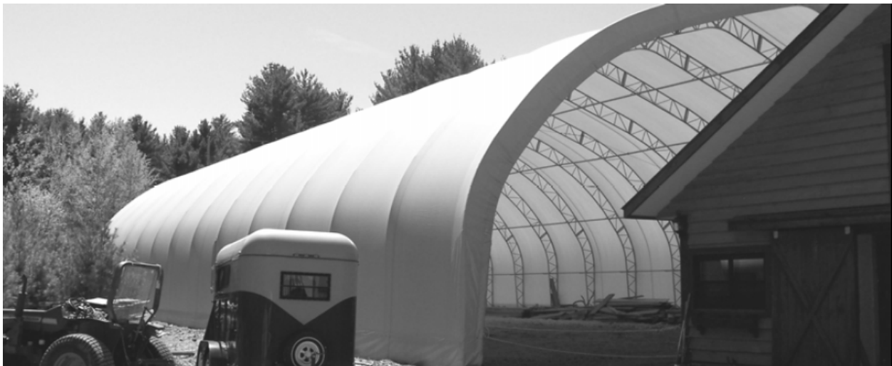
Figure 2: Image of the structure over horse arena originally constructed without a permit
